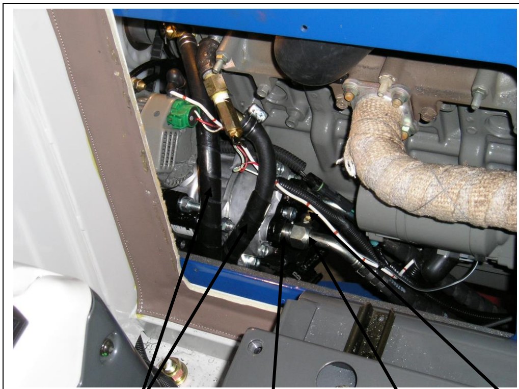
Heater hoses reconnected.
